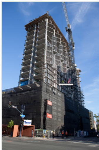
Celadon, located at Ninth Avenue and Broadway, is planned to mix 4,500 square feet of retail space, 4,000 square feet of office space and 250 affordable housing units.
